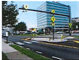
A mid-block crossing at Presidential Blvd., a busy road in Lower Merion Township, has a pedestrian refuge island and rapid flashing beacons for improved visibility.
